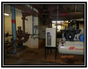
We currently have 3 diagram air pumps that run 24hrs a day which provide pumping for the thickeners and the digesters. The air is supplied by air compressors which also run constantly. The compressor is reaching the end of its service life and is becoming a high maintenance item and is costly. Currently by switching over to the new style pumps it will cut down on the electrical consumption, spare parts on hand for the pumps and compressor. All work on the new pumps can be done in-house.
