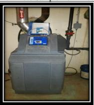
The current sampler is going on 15yrs old and we have had issues with the refrigeration unit. Even though it is still working the plan is to replace with a new unit and keep this unit as a backup for the other samplers in the facility. We have 5 of these samplers thru out the plant.
